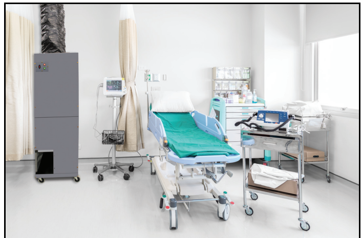
Fig. 2 – Room Setup Example for Negative Air
